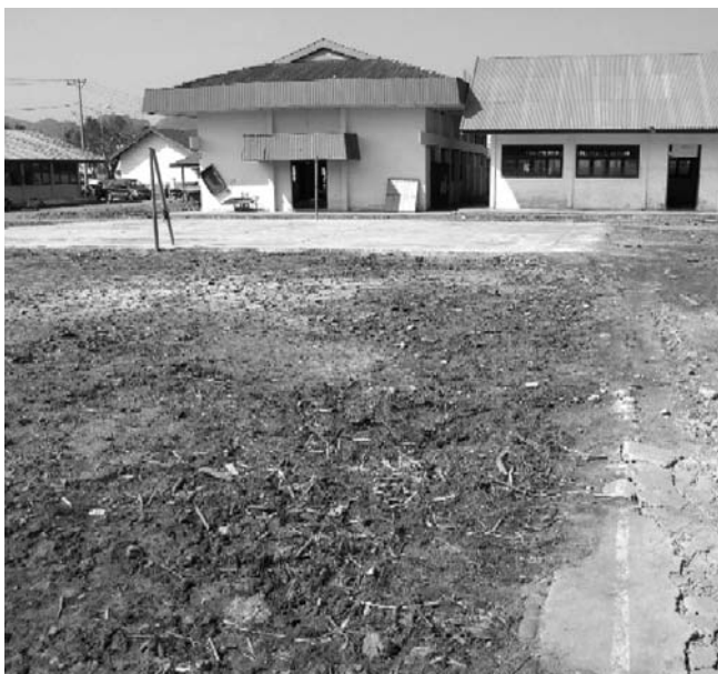
Repaired secondary school MAN2 in Indonesia
